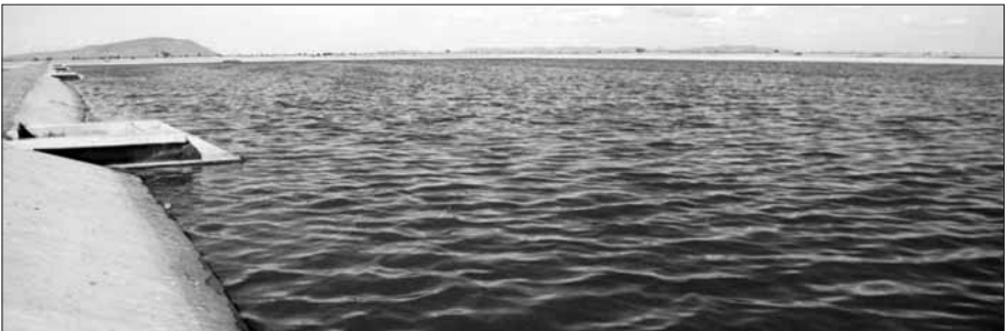
Figure 9.1 One of Phase II 21-ha Primary Facultative Ponds at Dandora, Nairobi, Kenya
